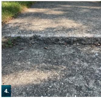
Different types of problem areas you may encounter: Downspouts that discharge over sidewalks (1 and 2), uneven sidewalk tiles (3), and poor drainage or low spots in parking lots may lead to over salting due to ice forming on surfaces (4).
