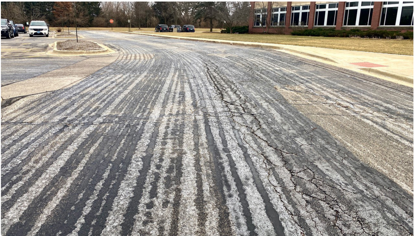
An example of good anti-icing application in a parking lot, note the wet/dry spray pattern.
